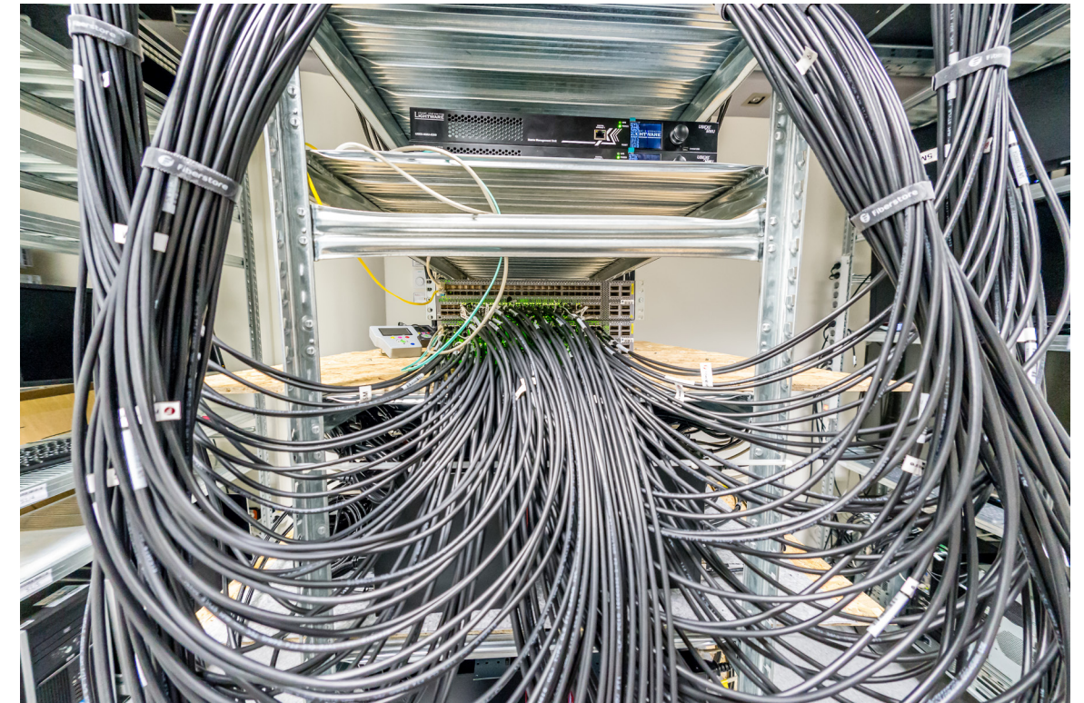
Hundreds of DAC cables run into the Juniper switches in the 24/7 testing room
